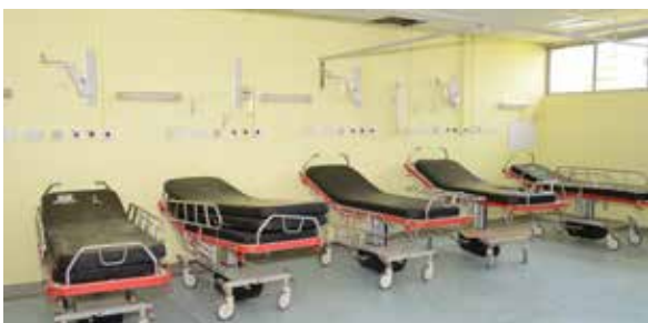
The casualty section completely renovated
