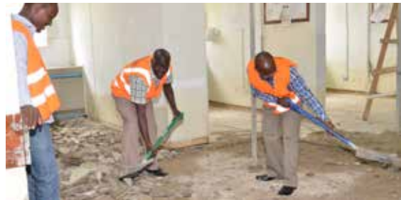
The reconstruction work for the floor begins
