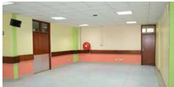
The floor redone and wall repainted
