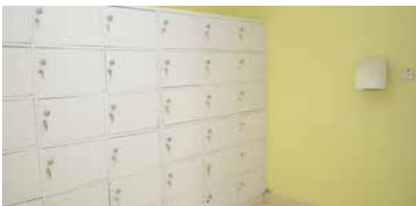
Staff locker room well done
