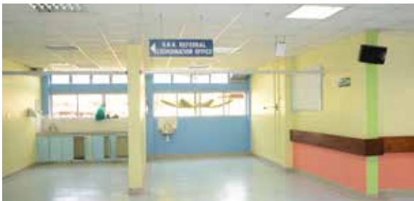
The floor and sink area renovated
